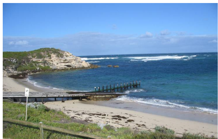
Figure 10: Gnarabup boat ramp / jetty
